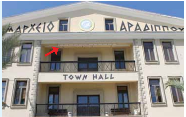
The municipality in the town of Aradippou, Cyprus, has already had nesting boxes for swifts placed on the front of its building following consultation with Amnon Hahn from Israel (the red arrow points to the nests); hundreds of Israeli couples are married in a civil ceremony in this municipality building (Photo: Elena Markitani)
